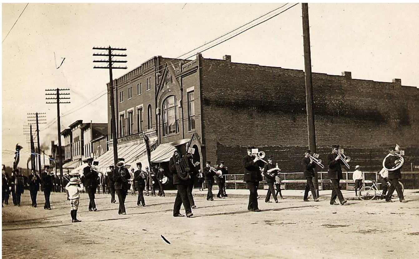
East Side of the 400 Block of South Stephenson Avenue, Facing North, Iron Mountain, ca. 1909: The northeast corner of the intersection of South Stephenson Avenue and East A Street was vacant for many years following the fire which burned the Flanagan Block to the ground February 25, 1904. There was an ice rink at this corner at times prior to the construction of the United States National Bank in 1921. The building with the triangular peak was the Odd Fellows Block, erected in about 1888. The M. Levy Company Store, one of the two larger department stores in Iron Mountain at this time, was north of the Odd Fellows Block. This postcard view was postmarked in Iron Mountain on July 23, 1909. [William John Cummings]
